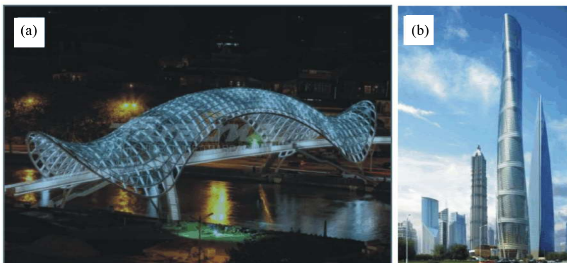
Fig. 2: Example of application of cold-bent glass panels in a HP shape: (a) Tbilisi Bridge of Peace, Tbilisi (Georgia), 2010 and (b) Shanghai Tower by Gensler, Shanghai (China), 2015
