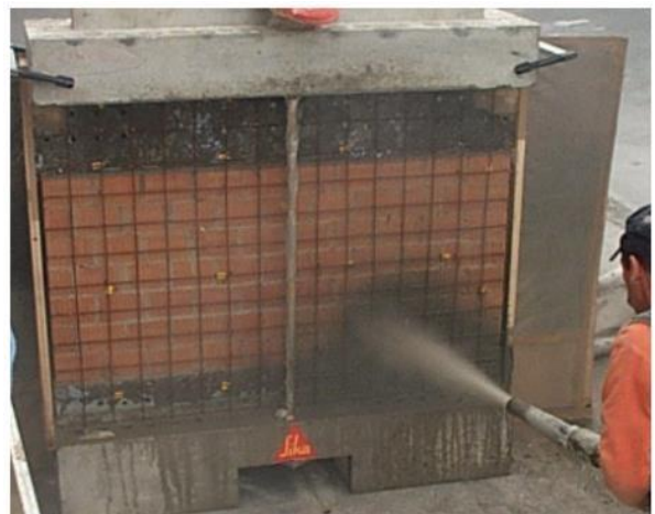
Fig. 7: Shotcrete spraying process (Wang et al. , 2018)
