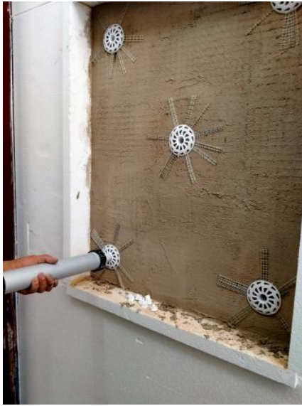
Fig. 11: Mortar injection in the diatons cavity
